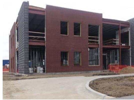
dow masonry, a tight seal required a bit of precision in materials and workmanship. “To meet the new UBC building code, walls have to have a complete thermal break, so we needed a masonry cavity insulation. We chose ACH Foam Technologies for several reasons,” continues Calacci. “Of course, they are local, about 30 miles from here, but their products also come in a wide range of thicknesses, which really helped us fill in around some complex architectural detailing.”
