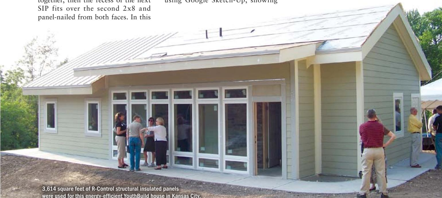
3,614 square feet of R-Control structural insulated panels were used for this energy-efficient YouthBuild house in Kansas City.
