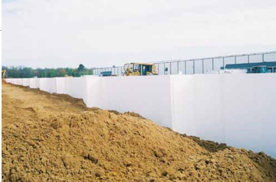
Over half a million board feet of Foam-Control Plus+ architectural grade perimeter and underslab insulation were used in the construction of the new cold storage facility.
