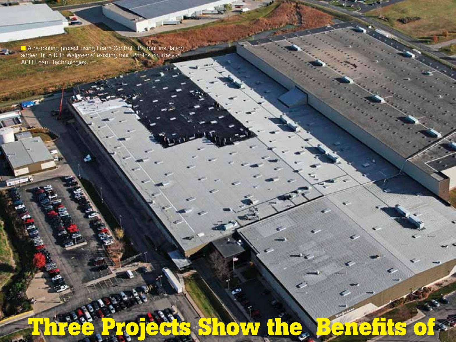
■ A re-roofing project using Foam Control EPS roof insulation added 16.5 R to Walgreens' existing roof. Photos courtesy of ACH Foam Technologies.
