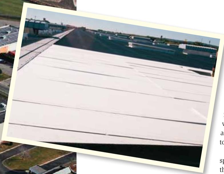
■ The Walgreens project used 1,175,625 board feet of 25psi Type IX Foam-Control® EPS Angle Cut Flute Filler Panels from ACH Foam Technologies.
