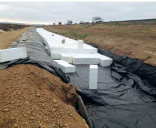
Prior to placing the geofoam blocks, the trench was lined with a gas-resistant membrane that protects the geofoam from oil and gas contaminants in roadway runoff.
