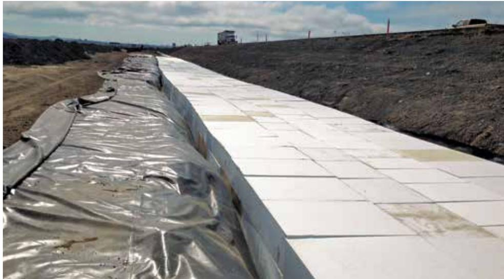
With the geofam blocks assembled into their final configuration, a gas-resistant membrane is set to be pulled over the top and fused together.
