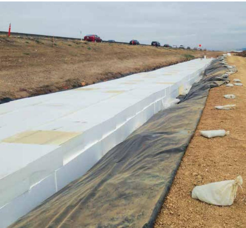
The geofoam will support the desired slope transition to mimic a natural wetlands embankment without threatening the long-term stability of adjacent Highway 37.
