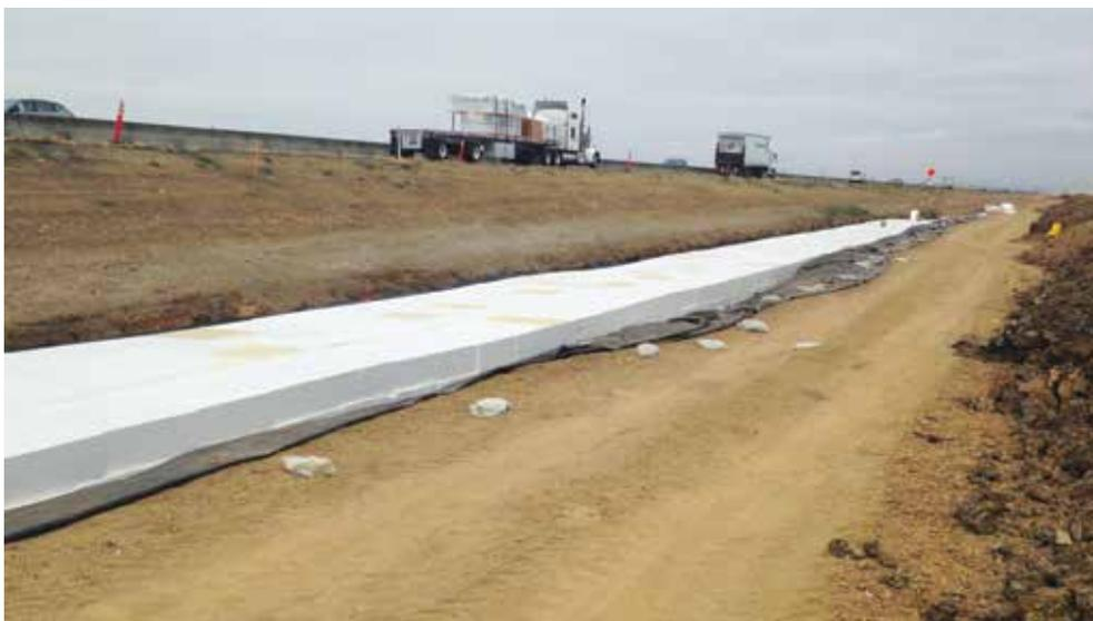
With a high compressive strength of 18.6psi at 1% deformation, the geofoam is about 1% of the weight of the soil fill.
