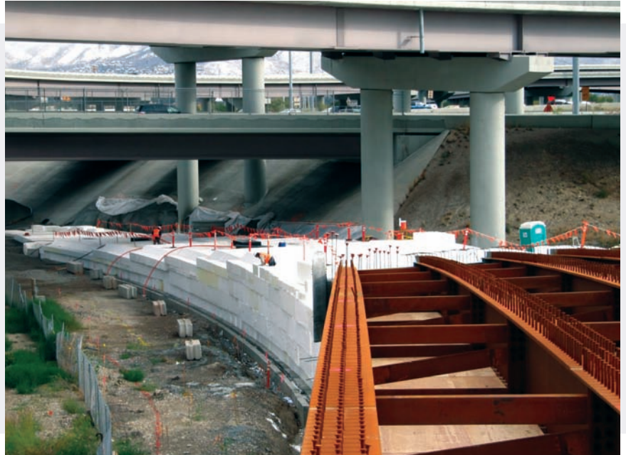
Seven areas along the West Valley TRAX line required the use ACH Foam Technologies' EPS geofoam.
